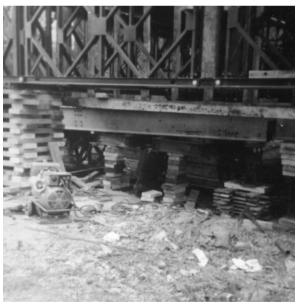
As time went by the barn was jacked higher and higher until the wheels could be moved under the barn and secured to a frame of large steel 'I' section joists which were fixed under the Bailey sections. There was also a scaffolding support framework inside the barn.
